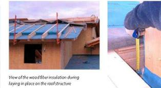
View of the wood fiber insulation during laying in place on the roof structure
