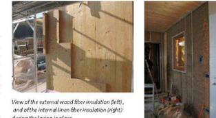
View of the external wood fiber insulation (left), and of the internal linen fiber insulation (right) during the laying in place
